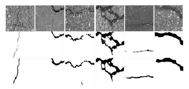
Figure 4: Prediction Results of U-Net<sub>Crack500</sub> on Crack500 Data (1<sup>st</sup> Row – Original Images, 2<sup>nd</sup> Row – Ground Truth, and 3<sup>rd</sup> Row - Predictions)
