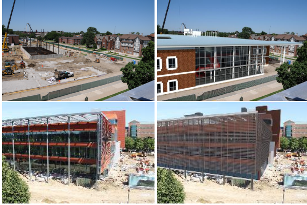
Figure 6.5: Our software automatically renders and composites photorealistic visualizations of the building model into in-progress construction photos. Original photos on left, visualizations on right.
