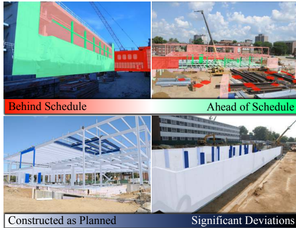
Figure 6.7: Construction photos can be annotated using a palette of smart-selection tools, indicating which regions/building components need review or are behind or ahead of schedule. Annotations are automatically transferred among all views (including those at previous/future dates), allowing field engineers and project managers to collaborate and save time in creating visualizations.
