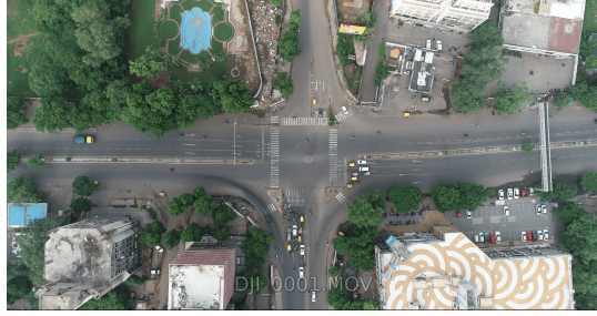
(b) Nehru bridge - Ashram road (N)
