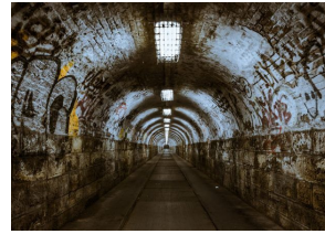
photo of an abandoned tunnel
