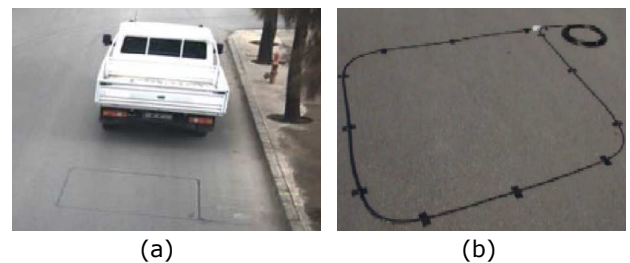
FIGURE 2. Types of loop detectors: (a) saw-cut loop [20]; (b) preformed loop [48].
