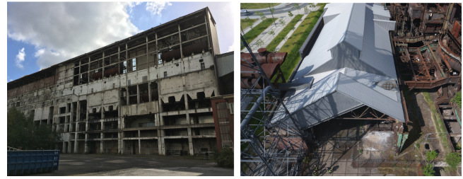
Figure 13. Buildings of the Gustav Knepper powerplant (left) and the Phoenix-West foundry (right).
