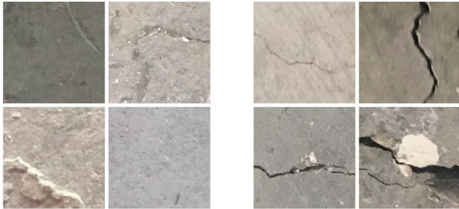
Fig. 3: Images from the CRACK data set [16]: negative (left) and positive (right) samples.
