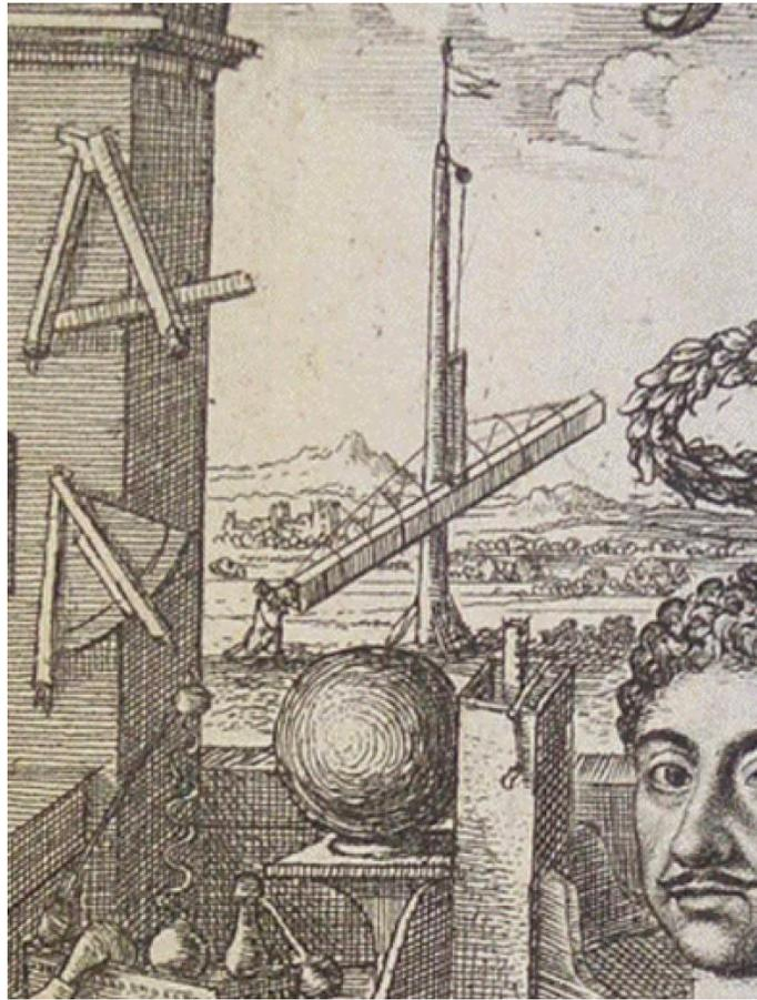
Robert Hooke's 60 foot telescope of 1666, from the frontispiece to Thomas Sprat's 1667 *History of the Royal Society of London*, engraving designed by John Evelyn; this telescope is hanging from the mast erected in 1658 for the 35 foot telescope. This fascinating engraving is so significant that it is the subject of an entire book, *The Image of Restoration Science* by Michael Hunter, Routledge 2016.
