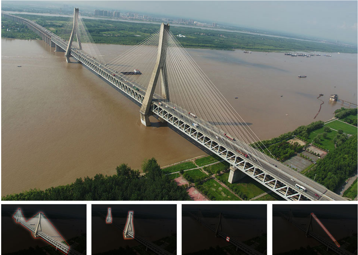
Figure 3: A picture of long-span cable-stayed bridge. Humans can delicately distinguish the bridge object in the picture from the background, then have information that this bridge has two towers arranged symmetrically, the truss blocks are aligned repeatedly and the cables are similar from one to another.
