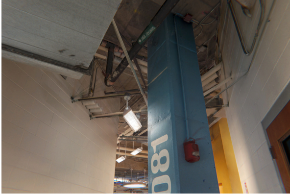
(a) Rendered image of the pipes and ventilation system in the basement.
