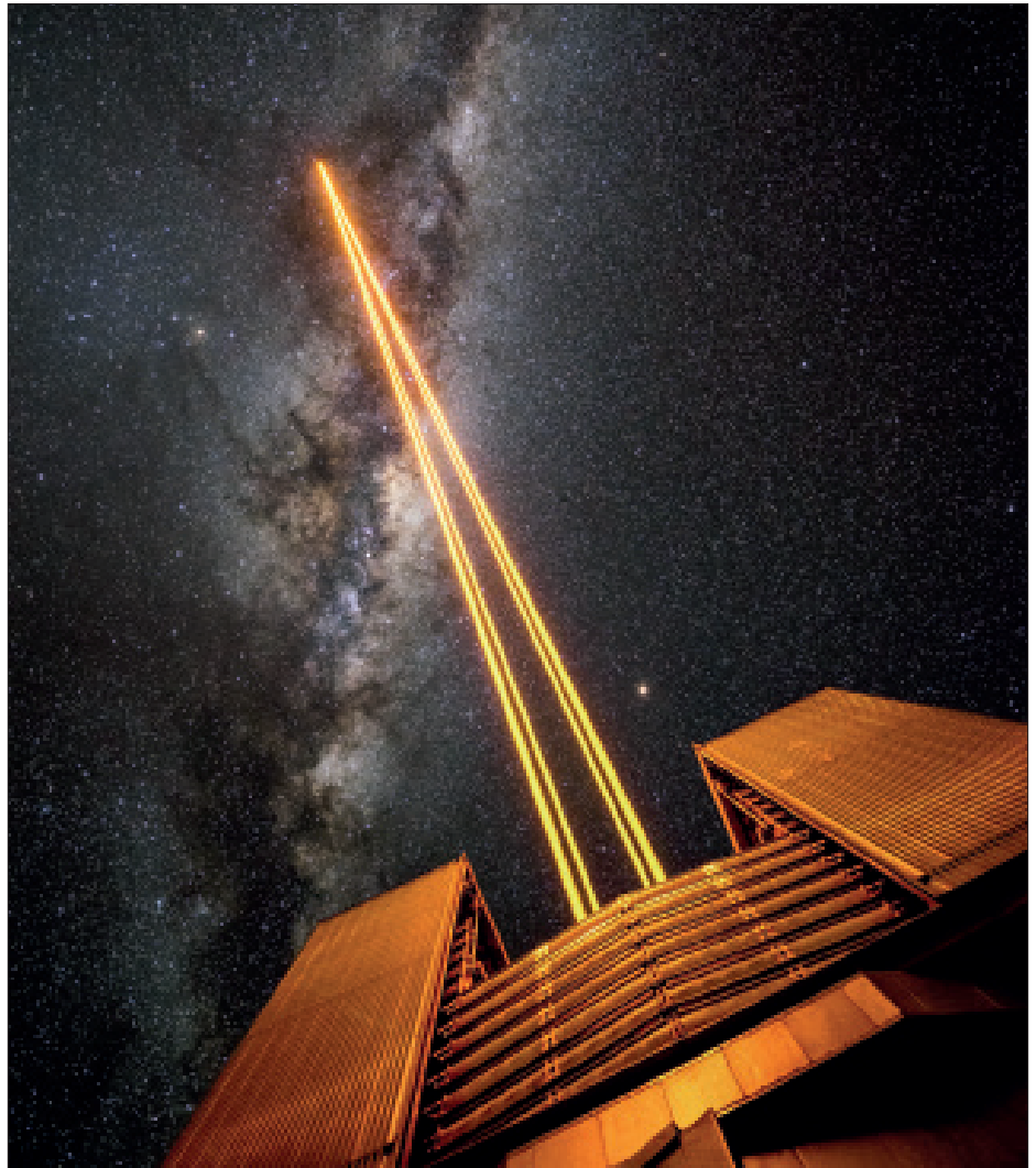
1 Four lasers create an artificial guide star from Unit Telescope 4 of ESO’s VLT at the Paranal Observatory, Chile. This is part of the VLT’s adaptive optics system, a technology which corrects the blurring effects of the Earth’s atmosphere to produce higher resolution images. (G Hüpdepohl [atacamaphoto.com]/ESO)
