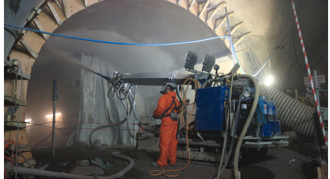
Fig. 1: Shotcrete application in a freshly excavated tunnel using a 5-DoF concrete spraying unit. Image provided by Costain Laing O'Rourke Joint Venture.
