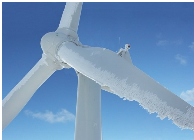
Figure 1: A photo of wind turbine's frozen blades [48].
