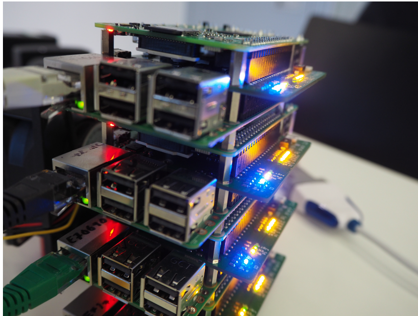
Figure 2: A micro data centre comprising a cluster of Raspberry Pis that was assembled at the University of Glasgow, UK. These data centres in contrast to large Cloud data centres are low cost and low power consuming.
