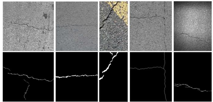
Fig. 3: Representative crack images (upper row) and ground truth (lower row) from five datasets.
