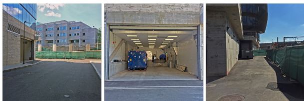
Fig. 7. Testing area: main street, loading dock and narrow street.
