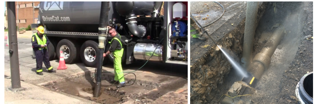
Figure 5: Using a hydrovac truck for inspection, requires a large truck and crew (left) and exposes the pipe material underground (right).
