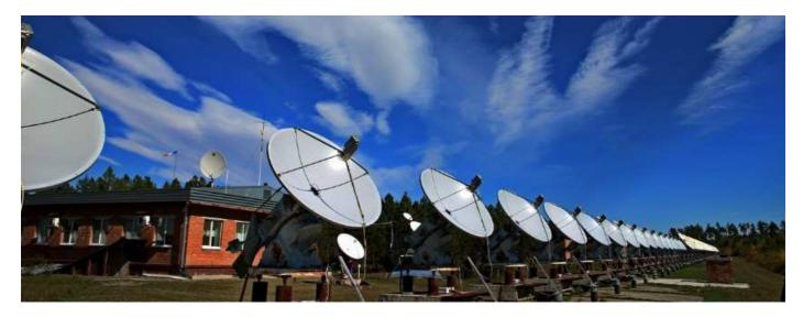
Figure 2: View of the 48-antenna SRH first stage (the east arm). White remote larger dishes on the right (east) belong to the old SSRT antenna system. Separate dishes on the ground behind the SRH antennas belong to the total-flux spectropolarimeters (Zhdanov and Zandanov, 2015). The receiver and control systems are located in the working building visible behind the SRH antennas on the left.
