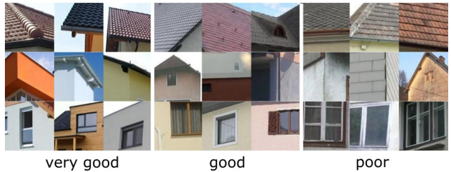
Figure 1: Visual appearance of the building elements roof (top row), facade (middle row), and window (bottom row) for the conditions very good, good, and poor.
