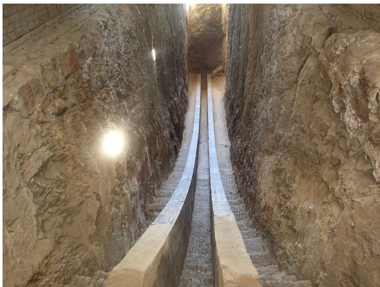
Left : Graduated low part of the double wall sextant. The two arcs are separated by 0,698 meter. The projected image of a star crossing the meridian moved from one wall to the other in exactly four minutes of time, which allowed the instrument to function also as a clock. Right : Sectional view of the Samarkand Observatory and its built-in quadrant.
