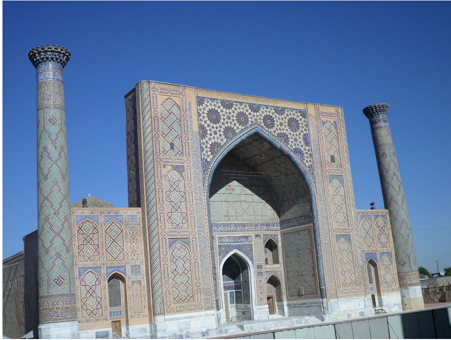
The madrasa built in Samarkand's Registan square under the reign of Ulugh Beg, between 1417 and 1420.
