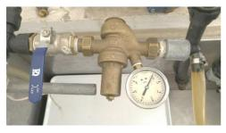
Figure 2. Shut-off valve, pressure regulator and pressure sensor (manometer).
