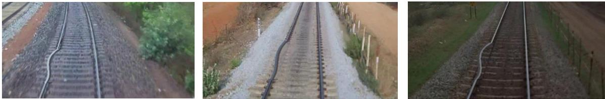
Figure 4 Examples of images simulated for sun kinks
