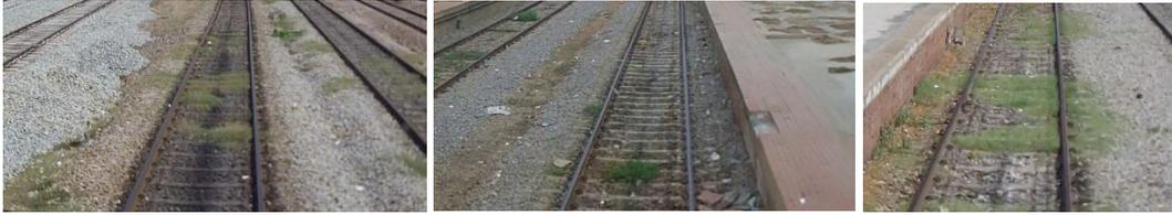
Figure 5 Vegetation overgrowth predicted correctly by the model
