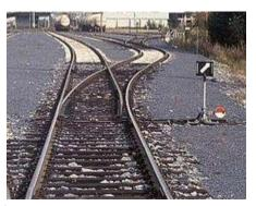
rails (the stock rails). These points can be moved laterally into one of two positions to direct a train coming from the point blades toward the straight path or the diverging path. A train moving from the narrow end toward the point blades (i.e. it will be directed to one of the two paths depending on the position of the points) is said to be executing a facing-point movement. Unless the switch is locked, a
