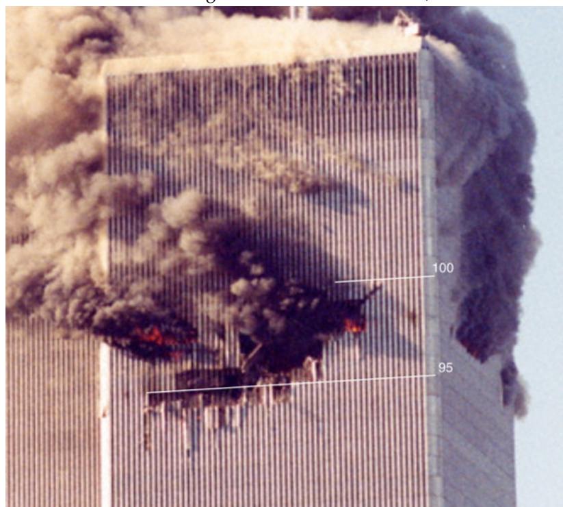
FIGURE 17. North side of the North Tower, [NIST, 2005c, p.35]. The white lines and the floor number are added on the basis of Figure 18.
