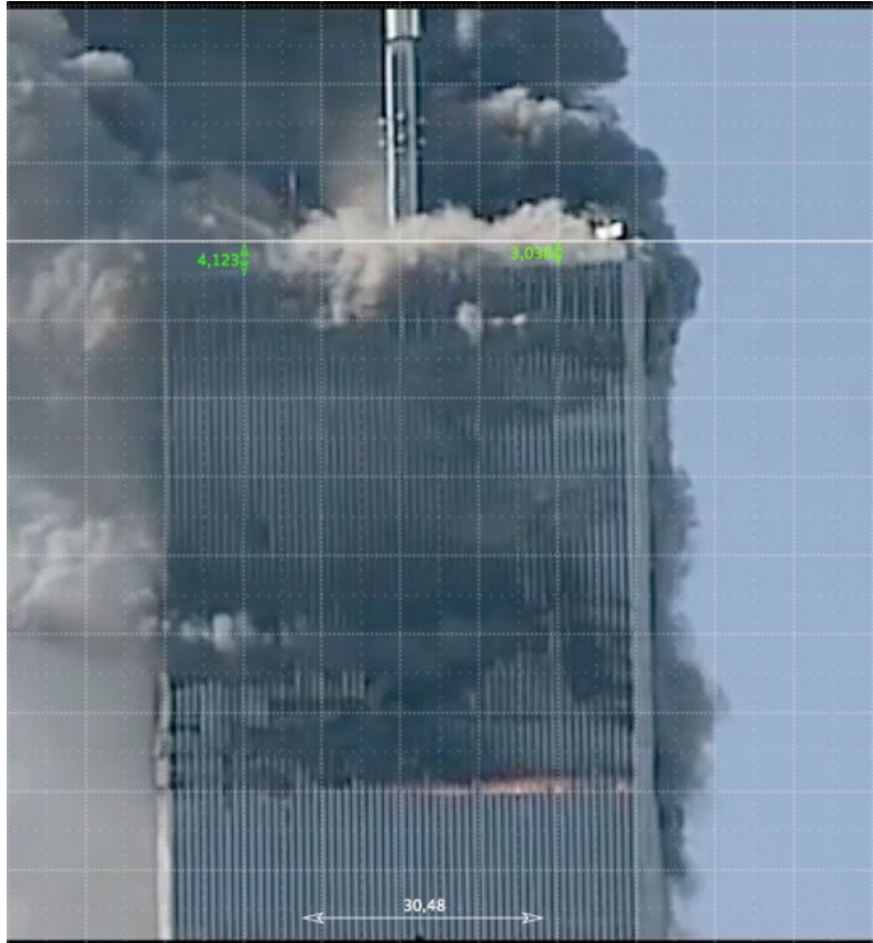
FIGURE 20. Measuring the position of the bottom of the roof at frame 934, t = 0 sec.
