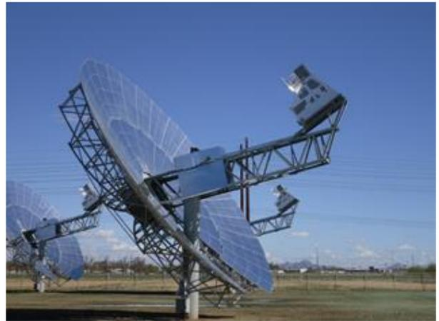
*Figure 1- Dish-Stirling engine Power plants*
