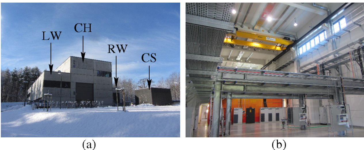
Fig. 1: The DRESHDYN building at HZDR. (a) External view, (b) interior of the central hall.
