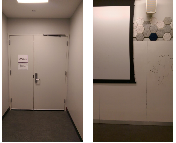
Fig. 4: Examples pictures of two different material types, a steel door (left) and a whiteboard writing wall (right). The whiteboard writing wall had a projector screen covering a portion of the surface as shown in the picture, however penetration through the screen was not measured.
