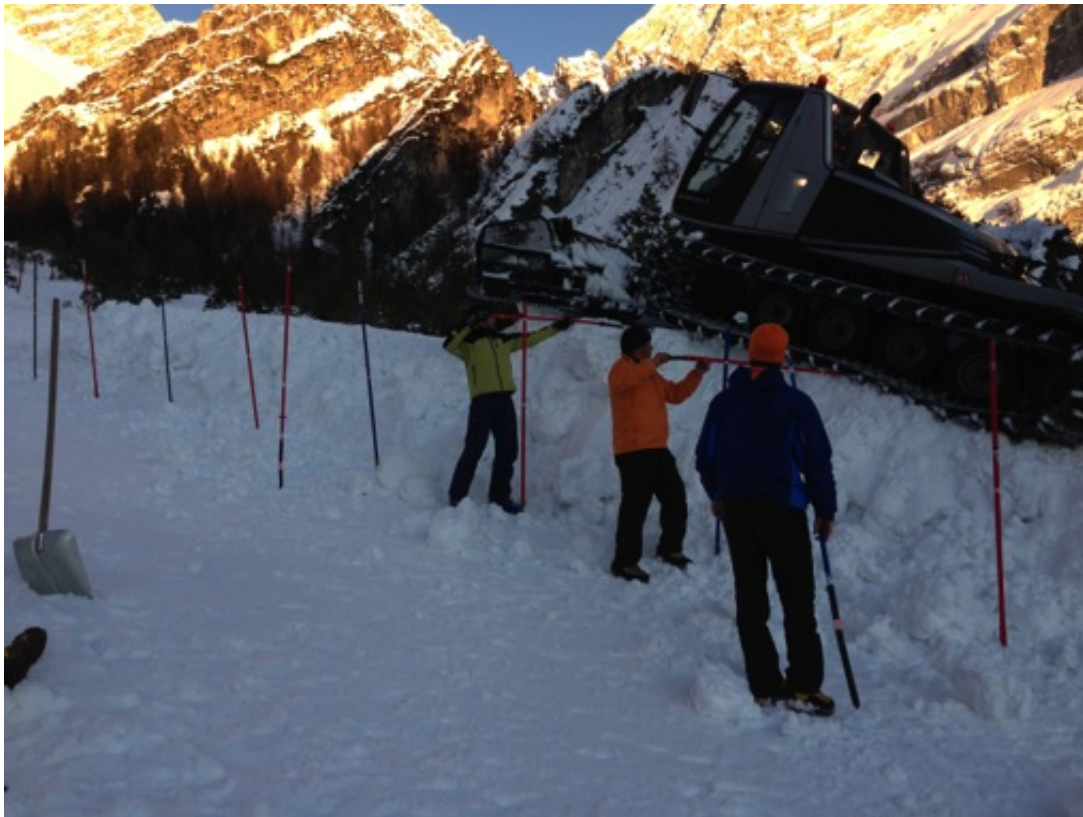
FIG. 1: In the process of constructing the constant EFH jump on the Antelao pitch of the San Vito ski resort.
