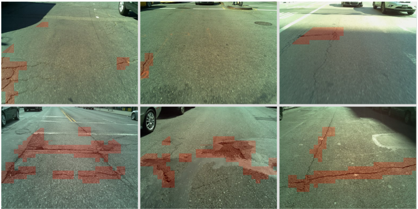
Figure 3: Crack detection results with defect regions highlighted in red.
