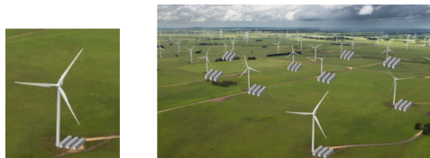
Fig. 1. ZCCloud containers below wind turbines. Turbines can be several MW, and wind farms >250 MW.
