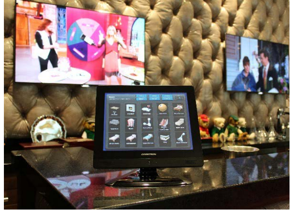
Figure 7. Crestron Touchpanel (Montgomery, 2013)
