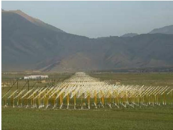
**Figure 1.** Photograph of the east-west baseline of the 21CMA, in which the building to the left is the control center.
