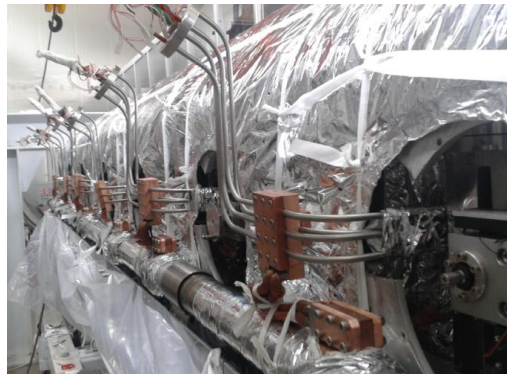
Fig. 8. Thermal anchors were connected to the anchor seats during the magnet assembly process, also as can be shown; the multilayer insulation was covered on the 5K cold shield.
