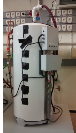
Fig. 1. Setup of the electric water heater used during the lab experiment. Eight temperature sensors were placed under the insulation material of the buffer tank.
