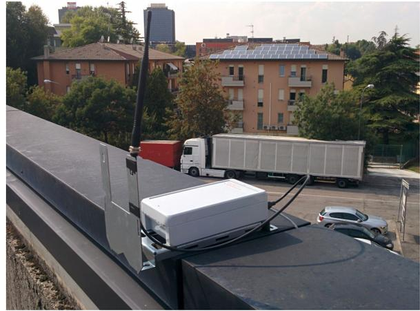
Fig. 3: LoRa™ gateway installation.
