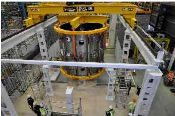
Fig. 2. MAST Vacuum Vessel being craned into its assembly area.
