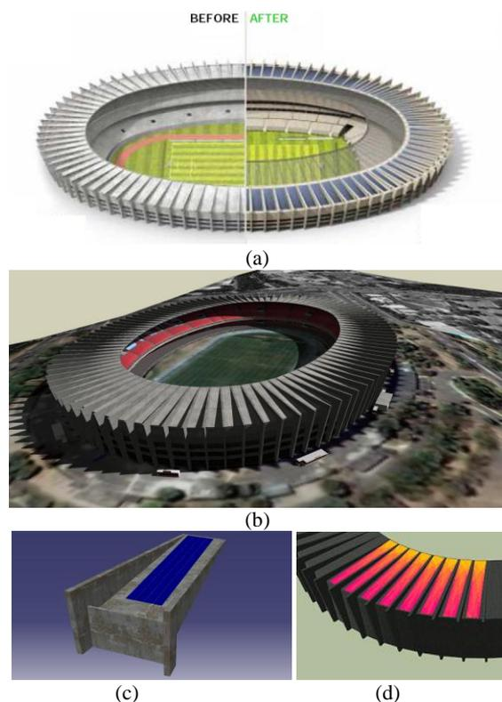
**Figure 8:** (a) The Mineirao stadium before and after the installation of the PV generator. (b) 3D model of the Mineirao stadium downloaded from the Google SketchUp 3D Warehouse library. (c) Closer view on one of the 88 PV generators. (d) Heat map of the shading affecting some of the PV generators.
