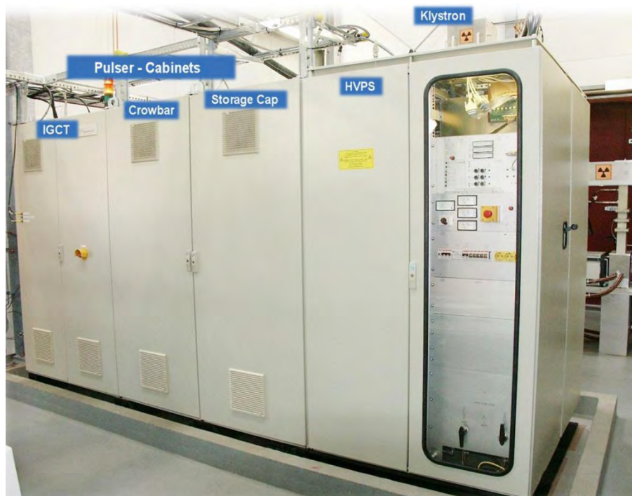
Figure 10.11. Klystron modulator built by PPT to operate the Thales TH1801, a 10 MW multi-beam klystron. The modulator consists of a capacitor bank using a series stack of IGCTs with bouncer droop compensation and pulse transformer matching of 1:12. It can switch a 12 kV pulsed voltage and 2 kA pulsed current. The pulse width can be varied from 50 \mu\text{s} to 2 ms. [[10.19]; Adapted under Creative Common Attribution 3.0 License ( www.creativecommons.org/licenses/by/3.0/us/ ) at www.JACoW.org .]
