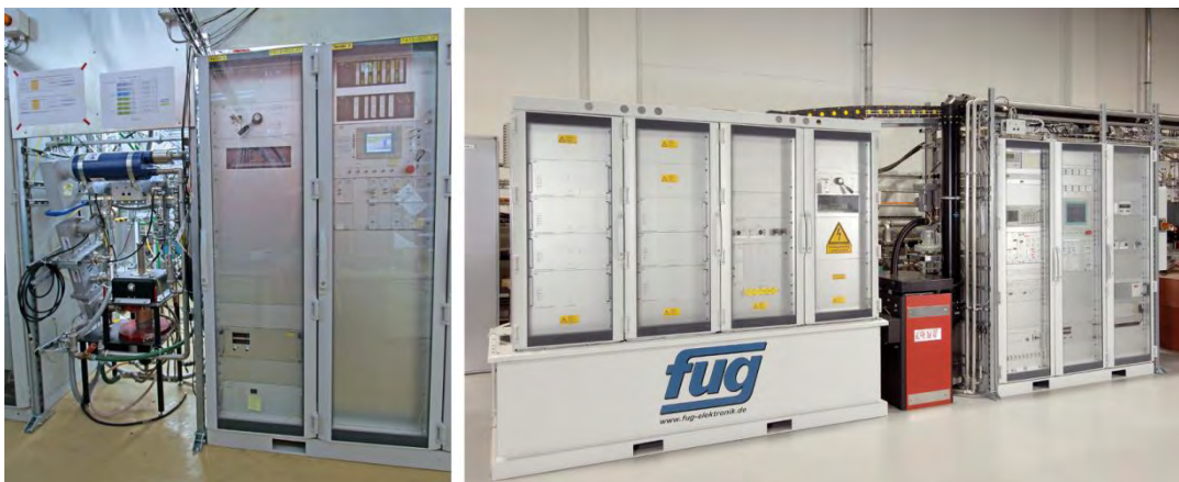
Figure 10.9. Example of two IOT based transmitters. On the left is a 30 kW, 1.3 GHz system operated at the HoBiCaT facility at the Helmholtz-Zentrum Berlin. On the right is an 80 kW, 500 MHz transmitter operated at the MLS. [[10.15]; Adapted under Creative Commons Attribution 3.0 License ( www.creativecommons.org/licenses/by/3.0/us/ ) at www.JACoW.org .]
