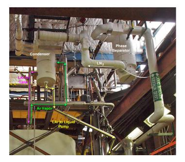
**Figure 5.** A photograph of the LAPD phase separator and condenser. The argon vapor path to the condenser and the two liquefied argon return paths are shown.
