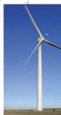
Medicine Bow, Clipper 2.5MW 93m Rotor
