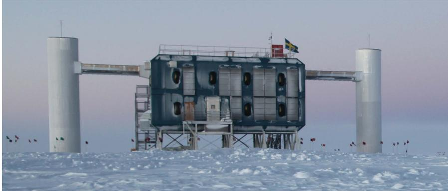
Figure 1: The IceCube Laboratory building houses power, communications and data acquisition systems for IceCube and other experiments at the South Pole (photo by S. Lidström/NSF).
