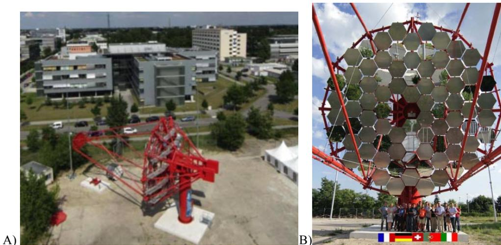
Fig. 17. The MST prototype installed in the DESY campus (Berlin). A) An aerial view of the telescope. B) the primary mirrors where part of the faced are dummy reflectors and part fully representative mirror tiles.
