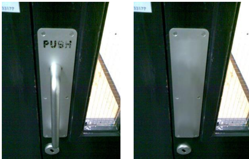
Fig. 2 A poorly designed door (left), and a well-designed door (right). Both doors require a push. Image on left used with permission (Walsh, 2007)
