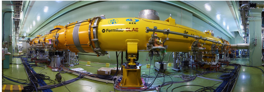
Figure 3.10 Fish-eye view of the S1-Global cryomodule at KEK.
