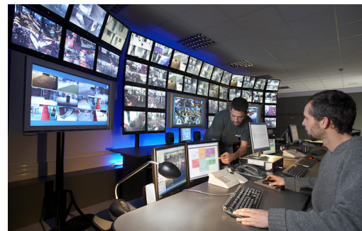
Figure 2. A control room for video surveillance (source [30])
