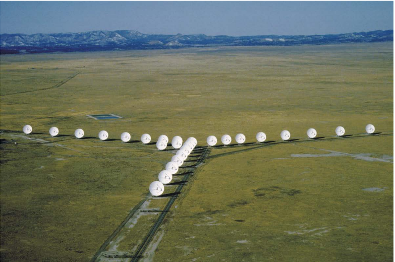
Figure 1. The Karl G. Jansky Very Large Array (VLA) located in central New Mexico includes twenty seven 25 meter antennas operating from a few hundred MHz to 50 GHz. Each antenna moves on railroad tracts along three arms to cover configurations ranging from 1 to 36 km. The angular resolution at the shortest wavelength and in the largest configuration is 0.04 arcseconds, about that of the Hubble Space Telescope.
