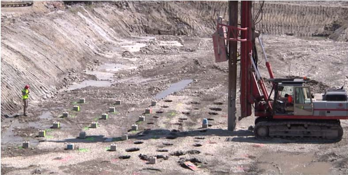
Fig. S1-2. Photograph of the seismic metamaterial experiment from the Ménard company.
