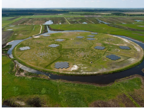
FIGURE 4. Aerial view of the LOFAR core. The island, called the superterp contains 6 of the 24 core stations. It is divided in larger and smaller patches which house the LBA and HBA antennas respectively.
