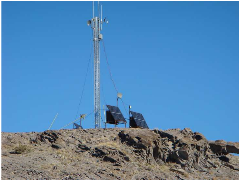
Figure 5: The Smelter Knolls communication tower, one of three in the array. There are three stands each with four solar panels. Those stands contain batteries, data acquisition PC and network instruments for long distance link.
