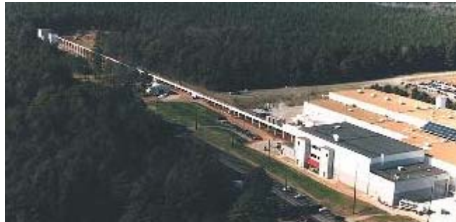
Figure 7. The X-Ray Calibration Facility at NASA's Marshall Space Flight Center. The small building to the far left houses the X-ray Source System including x-ray generators, monochrometers, and filters; the large building to the near right houses the instrument chamber. The distance from the XSS to the location of the entrance aperture of the telescope in the instrument chamber was 525-m facilitating simulating point sources.
